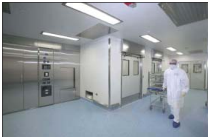
Finished preparation area.
