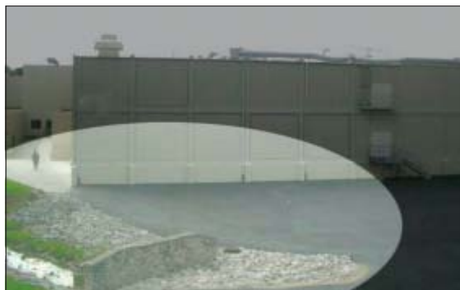
To avoid environmental impact, electric and gas utilities were tunneled under the creek.
