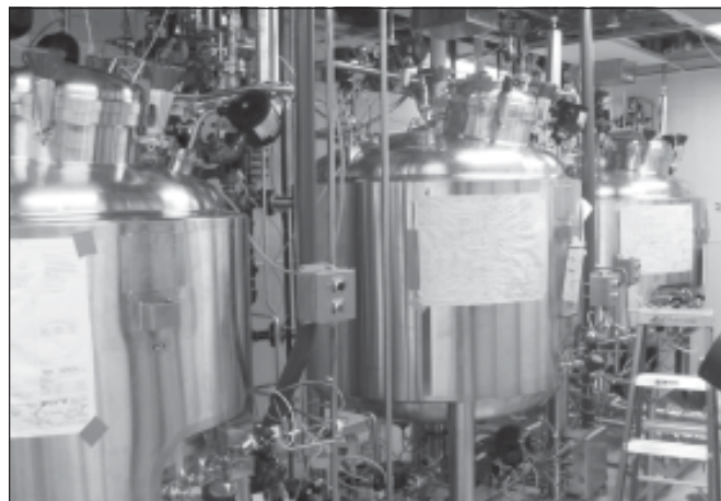
Figure 3. Field piping and tanks in purification buffer hold, during construction.
