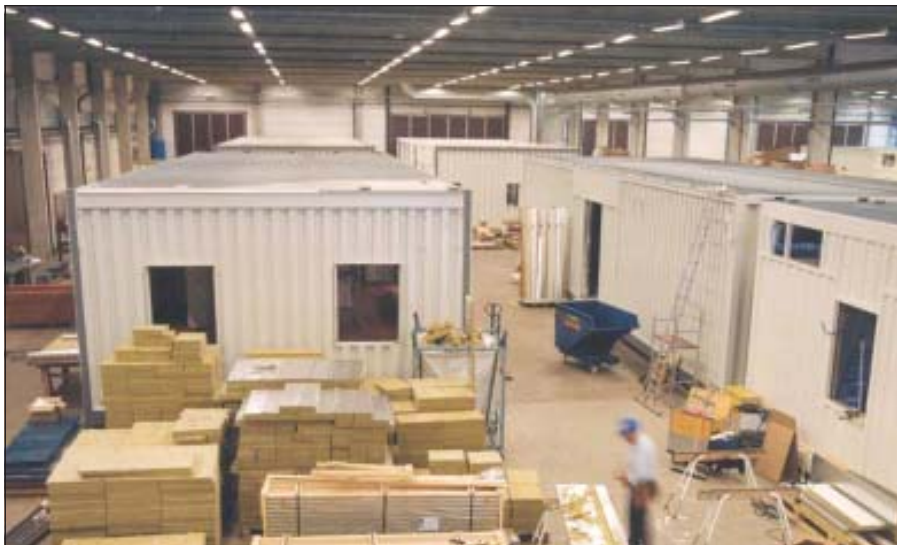
Facility modules built in a workshop environment.
