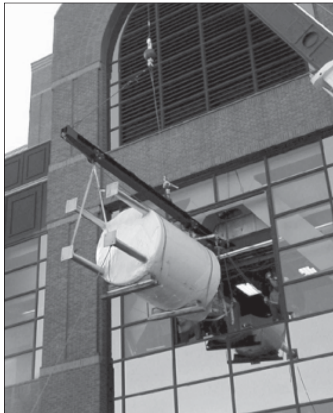
Figure 4. Tank rigging through second floor window.
