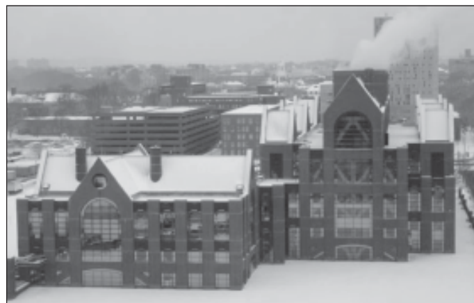
Figure 1. Genzyme's Allston, Massachusetts facility.
