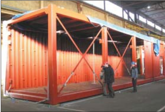
Module ready for outfitting and process equipment and utility installation.
